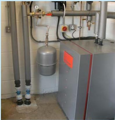
In compressing the vapour and condensing it, the heat is released. This heat is transferred (via a heat exchanger) to a hot water circulation system. The more compression, the higher the temperature becomes. So the final temperature of the output is, to a limit, up to us. Unfortunately, the higher we raise the temperature the less efficient the process becomes.
